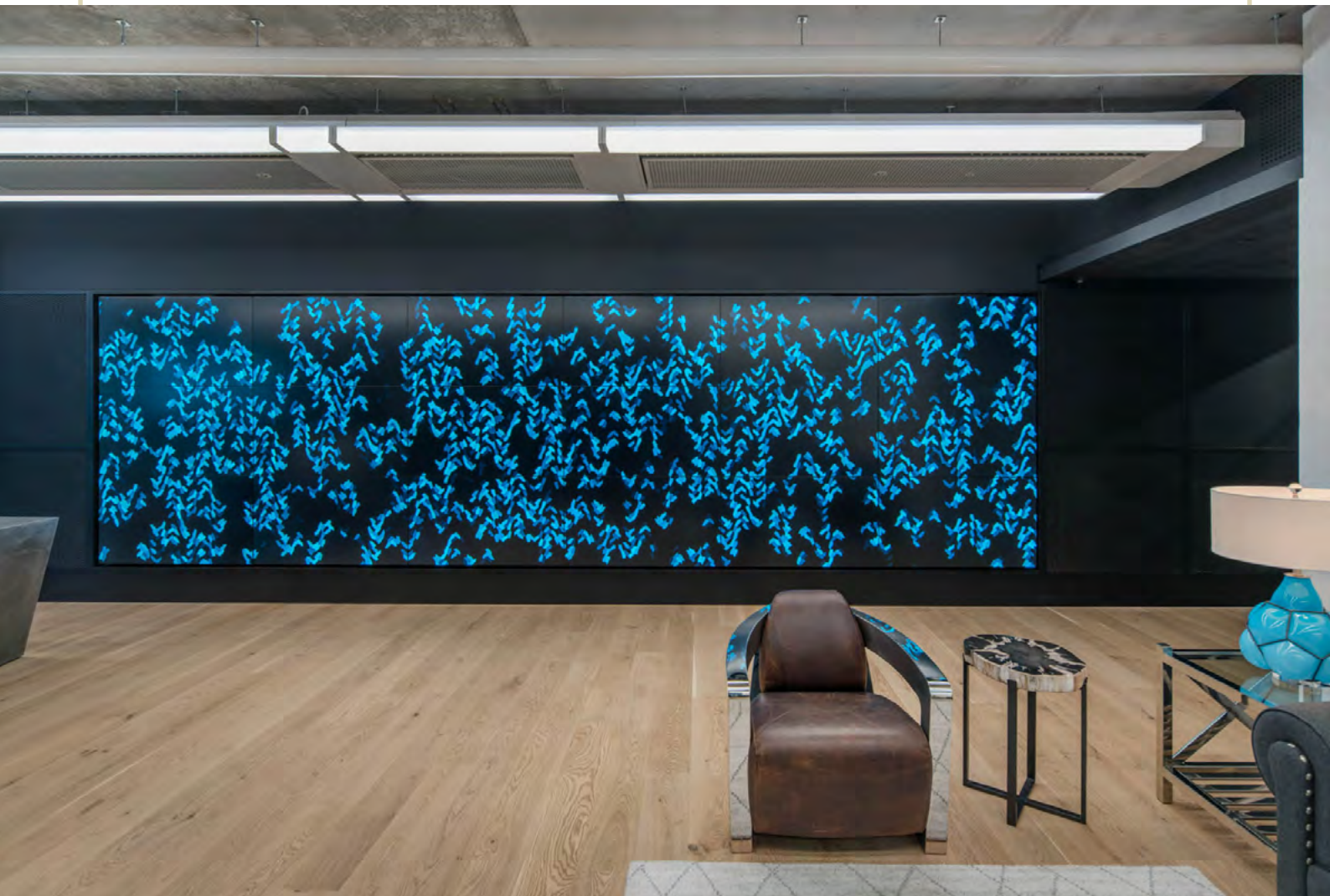
King Cross, Building R7 with Multi-Service Chilled Beams
