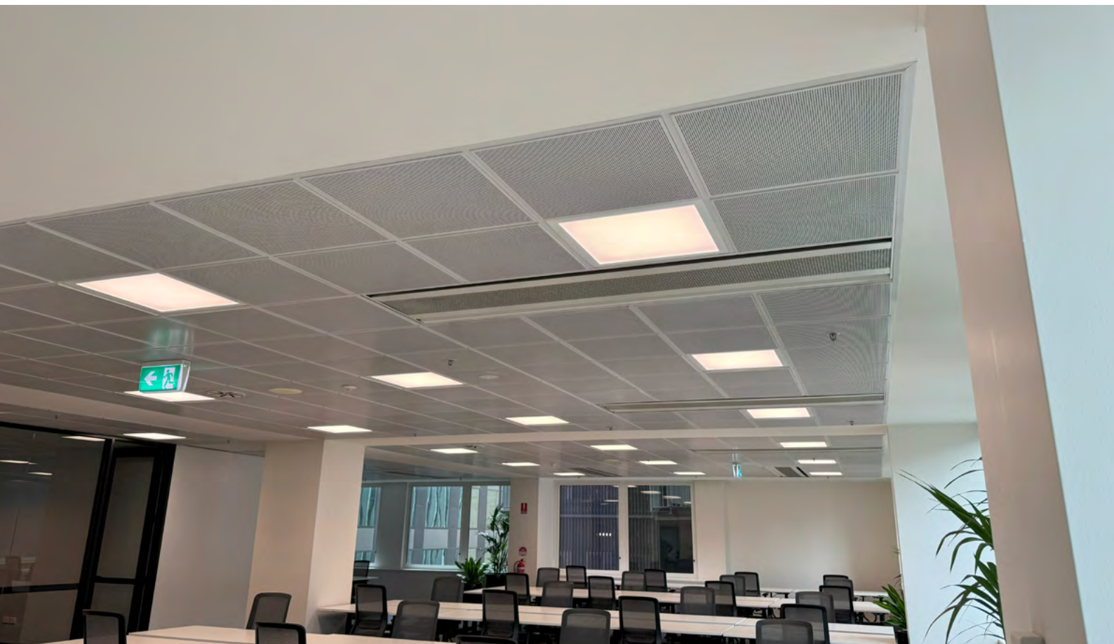
500 Collins Street photo - 2024
