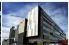
World Park Adelaide, Australia - 2011 Passive Chilled Beams
