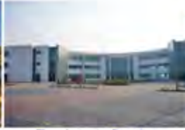
Business Centre Liverpool, UK - 2008 Active Chilled Beams
