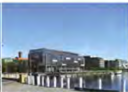
Google Headoffice Sydney, Australia - 2010 Passive Chilled Beams
