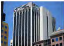
500 Collins Street Australia - 2010 Active Multiservice
