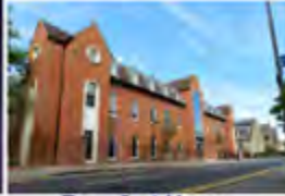
Beaufort House London, UK - 2012 Passive Multiservice
