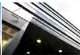
Bidborough House London, UK - 2008 Active Chilled Beams
