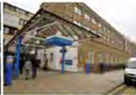
Great Ormond Street Hospital London, UK - 2015 Active Chilled Beams
