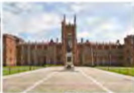
Queens University Belfast, UK - 2015 Passive Chilled Beams
