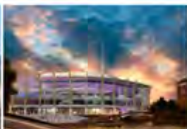
Barclaycard Arena Birmingham, UK - 2014 Passive Chilled Beams
