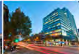
City Central Tower Adelaide, Australia - 2005 Passive Chilled Beams
