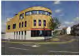
Walthamstow Station Walthamstow, UK - 2011 Passive Chilled Beams
