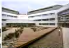
Cheshire Police Cheshire, UK - 2009 Active Chilled Beams
