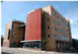
Liverpool College Liverpool, UK - 2010 Active Chilled Beams
