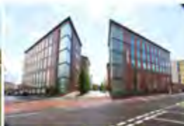
Langley Point Birmingham, UK - 2012 Passive Chilled Beams
