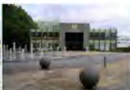
Coventry University Coventry, UK - 2008 Active Chilled Beams
