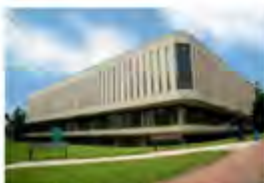
Hallward Library Nottingham, UK - 2008 Active Multiservice
