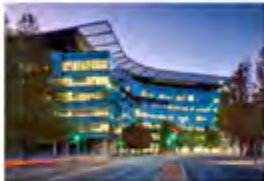
London Circuit Canberra, Australia - 2006 Passive Chilled Beams
