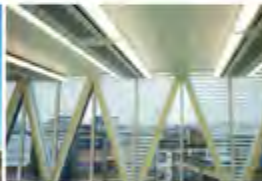
65 Southwark Street London, UK - 2012 Active Multiservice
