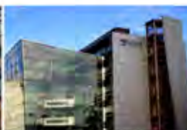
Suffolk County Council Suffolk, UK - 2008 Passive Chilled Beams
