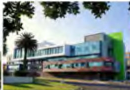
Warrambool Hospital Australia - 2009 Active Chilled Beams
