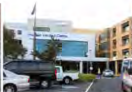
Monash Children's Hospital Australia - 2014 Active Chilled Beams
