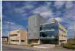
HDTI Coventry, UK - 2008 Active Chilled Beams
