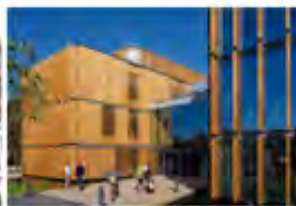
Alder Hay Research & Education Liverpool, UK - 2014 Active Chilled Beams
