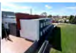
BBC Grafton House Middlesex, UK - 2012 Active Chilled Beams
