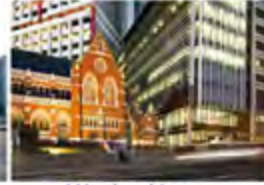
Wesley House Brisbane, Australia - 2008 Passive Chilled Beams
