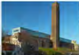
Tate Modern London, UK - 2012 Passive Chilled Beams
