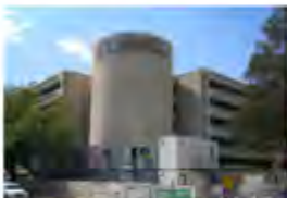
Edmund Barton Canberra, Australia - 2009 Active Chilled Beams
