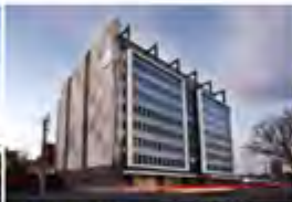
South Australia Police Adelaide, Australia - 2009 Passive Chilled Beams
