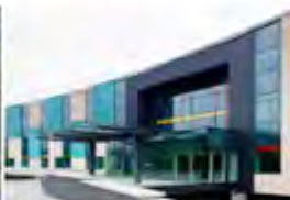
ACAD Hospitals - Stobhill Glasgow, UK - 2008 Active Chilled Beams
