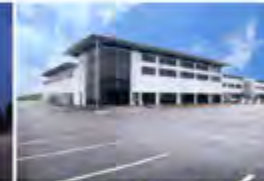
Project Vauxhall UK - 2006 Passive Chilled Beams
