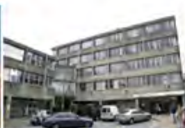
Northwick Park Hospital Harrow, UK - 2014 Active Chilled Beams
