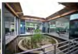
Vodafone Innovation South Africa - 2011 Passive Chilled Beams
