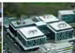
Telcom Square New Zealand - 2010 Passive Chilled Beams
