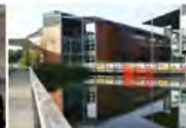
Vodafone London, UK - 2001 Passive Chilled Beams
