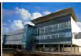
QMC Hospital Nottingham, UK - 2008 Active Chilled Beams
