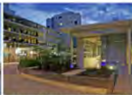
Royal Hobart Hospital Hobart, Tasmania - 2010 Active Chilled Beams
