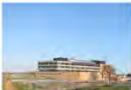
Cambridge Metallurgy Cambridge, UK - 2012 Passive Chilled Beams
