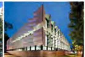
Belconnen Police Australia - 2010 Passive Chilled Beams
