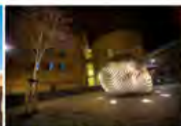
Cambridge Library Cambridge, UK - 2008 Active Chilled Beams
