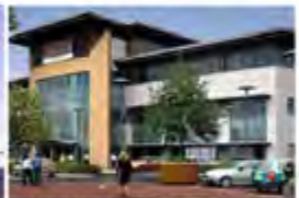
Veolia Environmental Cannock, UK - 2012 Passive Chilled Beams
