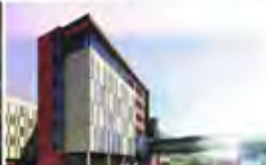
Skywalk Anchorage, Alaska - 2015 Active Multiservice
