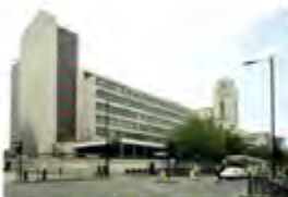
National Audit Office London, UK - 2005 Active Multiservice
