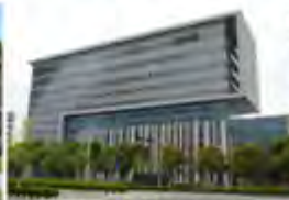
Monash University Australia - 2009 Active Chilled Beams
