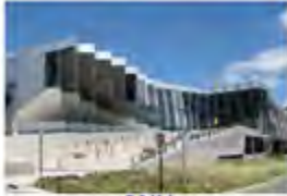
ANU Australia - 2013 Active Chilled Beams
