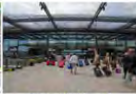
Gatwick Airport Gatwick, UK - 2015 Passive Chilled Beams
