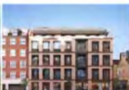
18-20 Grosvenor Street London, UK - 2014 Active Chilled Beams
