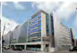
55 Baker Street London, UK - 2008 Active Multiservice
