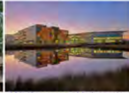
Wollongong University NSW, Australia - 2011 Passive Chilled Beams
