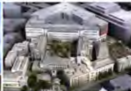
St Barts Hospital London, UK - 2009 Active Chilled Beams
