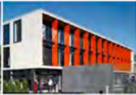
National Film & TV School Beaconsfield, UK - 2016 Active MSCB's & Chilled Beams
