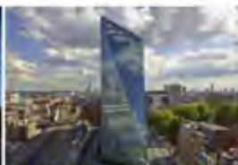
240 Blackfriars Road London, UK - 2014 Active Chilled Beams
