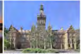
Melbourne University Australia - 2010 Active Chilled Beams
