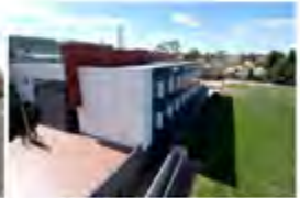
Trinity Grammer Trinidad & Tobago - 2012 Passive Chilled Beams
