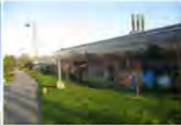
Exeter University Exeter, UK - 2012 Active Chilled Beams
