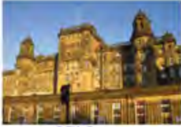
GRI Gynae Glasgow, UK - 2008 Active Chilled Beams
