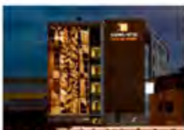
Sudima Hotel New Zealand - 2010 Active Chilled Beams
