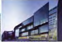
IMAS Hobart Australia - 2012 Passive Chilled Beams
