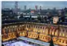
Kings College London, UK - 2009 Passive Chilled Beams
