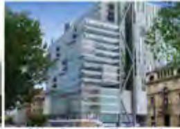
City Centre Tower 8 Australia - 2011 Passive Chilled Beams
