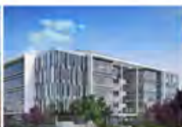
1 Canberra Avenue Australia - 2013 Passive Chilled Beams
