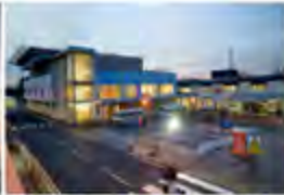
Frimley Park Hospital Frimley, UK - 2011 Active Chilled Beams
