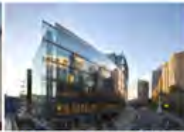
Kangan Batman Tafe Australia - 2010 Active & Passive Chilled Beams
