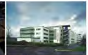
BT Leavesden Wafford - 2002 Passive Chilled Beams
