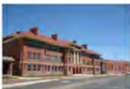
Trinidad School Trinidad & Tobago - 2011 Passive Chilled Beams
