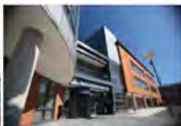
West Suffolk House Ipswich, UK - 2014 Passive Chilled Beams
