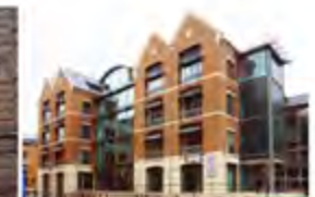
BT Nottingham Nottingham - 1998 Passive Chilled Beams
