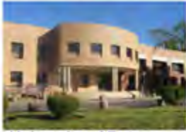
University of Botswana Botswana - 2011 Active Chilled Beams
