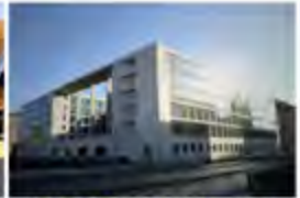
SIEC Tonsley House Australia - 2013 Active & Passive Chilled Beams
