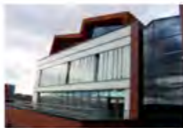
Charles Street, Sheffield University Sheffield, UK - 2015 Passive Chilled Beams
