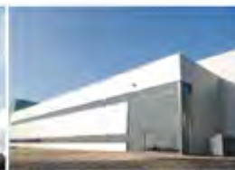
Kingswood Lakeside Cannock, UK - 2010 Passive Chilled Beams
