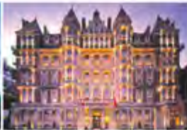
Knightsbridge Hotel London, UK - 2010 Passive Chilled Beams
