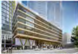
Barangaroo C2 Sydney, Australia - 2016 Passive Chilled Beams
