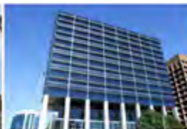
Sydney Water House Australia - 2008 Passive Chilled Beams
