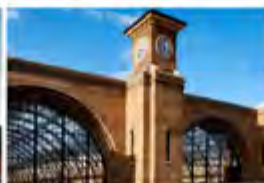
Kings Cross London, UK - 2008 Active Chilled Beams
