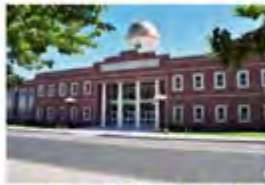
Ocean City School New Jersey, USA - 2015 Active Chilled Beams
