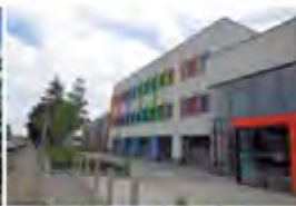
Northbrook College Worthing, UK - 2014 Active Multiservice
