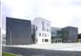
Loxford School London, UK - 2009 Active Chilled Beams
