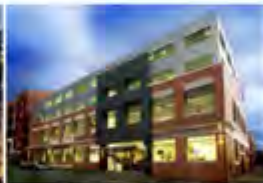
Batman Street Australia - 2009 Passive Chilled Beams
