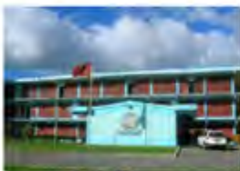
Five Rivers Trinidad - 2010 Passive Chilled Beams
