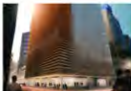
50 Flinders Street Adelaide, Australia - 2014 Passive Chilled Beams
