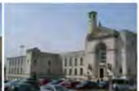
Southampton Civic Centre Southampton UK - 2011 Active Multiservice
