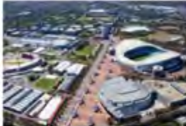
Sydney Olympic Park Sydney, Australia - 2007 Passive Chilled Beams
