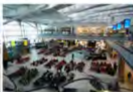
Gatwick Terminal London, UK - 2008 Passive Chilled Beams
