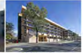
64 Allara Street Australia - 2007 Passive Chilled Beams
