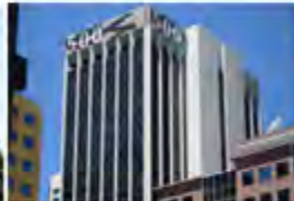
500 Collins Street Australia - 2005 Active Multiservice
