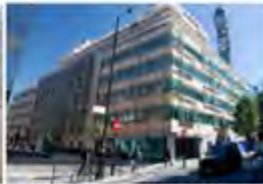
New Cavendish Street London, UK - 2009 Active Multiservice
