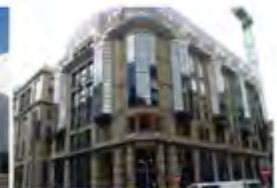
Meridian Court Edinburgh, UK - 2010 Active Chilled Beams
