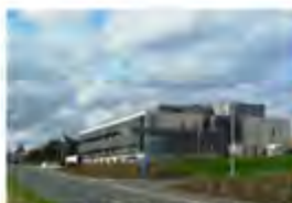
West Yorkshire Police Wakefield, UK - 2014 Passive Chilled Beams
