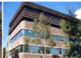
RMIT 9 Australia - 2010 Active Chilled Beams
