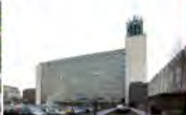
Newcastle Civic Centre Newcastle, UK - 2016 Active Chilled Beams
