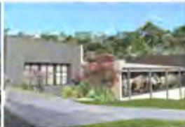
Kingston Aged Care Australia - 2009 Active Chilled Beams
