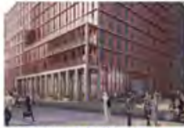
Building R7, King Cross London, UK - 2016/17 Active Multiservice
