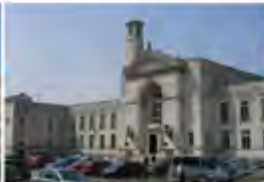
Civic Offices Southampton, UK - 2009 Active Chilled Beams
