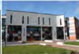
Stafford College Stafford, UK - 2012 Active Chilled Beams
