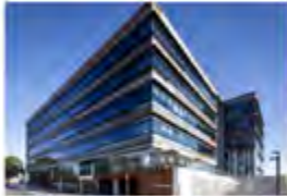
5 Murray Rose Avenue Sydney, Australia - 2012 Passive Chilled Beams
