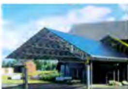
Wrexham A&E Wrexham, UK - 2008 Active Chilled Beams
