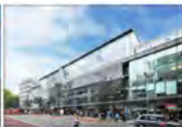
High Holborn London, UK - 2014 Active MSCB's & Chilled Beams
