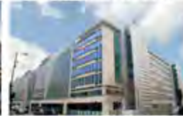
55 Baker Street London, UK - 2008 Active Multiservice
