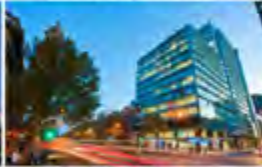
City Central Tower Adelaide, Australia - 2005 Passive Chilled Beams
