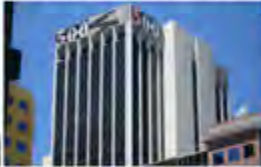
500 Collins Street Australia - 2005 Active Multiservice
