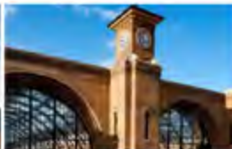
Kings Cross London, UK - 2008 Active Chilled Beams
