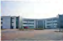
Business Centre Liverpool, UK - 2008 Active Chilled Beams
