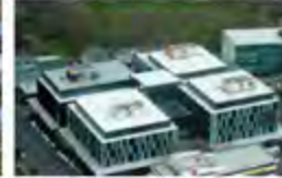
Telcom Square New Zealand - 2010 Passive Chilled Beams
