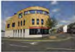
Walthamstow Station Walthamstow, UK - 2011 Passive Chilled Beams
