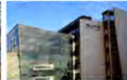
Suffolk County Council Suffolk, UK - 2008 Passive Chilled Beams
