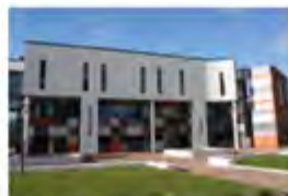
Stafford College Stafford, UK - 2012 Active Chilled Beams
