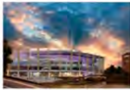
NIA Birmingham Birmingham, UK - 2014 Passive Chilled Beams
