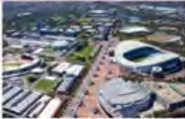
Sydney Olympic Park Sydney, Australia - 2007 Passive Chilled Beams
