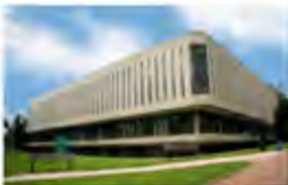
Hallward Library Nottingham, UK - 2008 Active Multiservice
