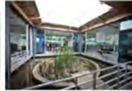
Vodafone Innovation South Africa - 2011 Passive Chilled Beams
