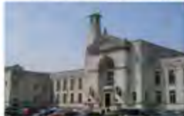
Civic Offices Southampton, UK - 2009 Active Chilled Beams
