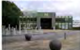
Coventry University Coventry, UK - 2008 Active Chilled Beams
