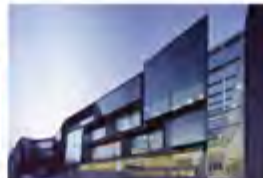
IMAS Hobart Australia - 2012 Passive Chilled Beams
