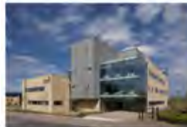
HDTI Coventry, UK - 2008 Active Chilled Beams
