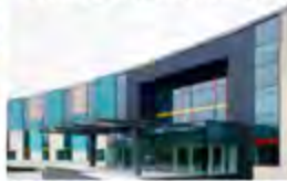
ACAD Hospitals - Stobhill Glasgow, UK - 2008 Active Chilled Beams
