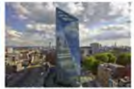
240 Blackfriars Road London, UK - 2014 Active Chilled Beams
