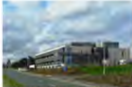
West Yorkshire Police Wakefield, UK - 2014 Passive Chilled Beams
