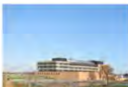
Cambridge Metallurgy Cambridge, UK - 2012 Passive Chilled Beams
