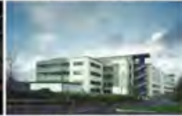
BT Leavesden Watford - 2002 Passive Chilled Beams
