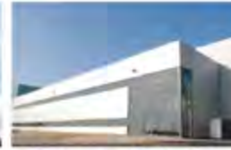
Kingswood Lakeside Cannock, UK - 2010 Passive Chilled Beams
