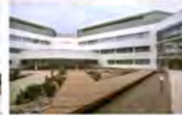
Cheshire Police Cheshire, UK - 2009 Active Chilled Beams
