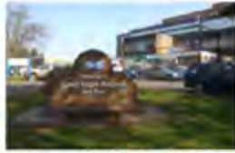
Good Hope Hospital Sutton, UK - 2010 Active Chilled Beams
