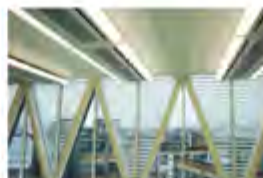
65 Southwark Street London, UK - 2012 Active Multiservice
