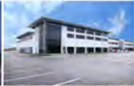
Project Vauxhall UK - 2006 Passive Chilled Beams
