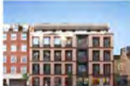
18-20 Grosvenor Street London, UK - 2014 Active Chilled Beams
