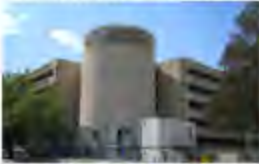
Edmund Barton Canberra, Australia - 2009 Active Chilled Beams
