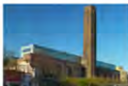
Tate Modern London, UK - 2012 Passive Chilled Beams
