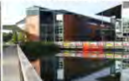
Vodafone London, UK - 2001 Passive Chilled Beams
