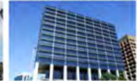
Sydney Water House Australia - 2008 Passive Chilled Beams
