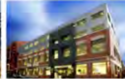
Batman Street Australia - 2009 Passive Chilled Beams
