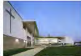
All Saints Academy Cheltenham, UK - 2011 Passive Chilled Beams
