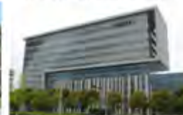
Monash University Australia - 2009 Active Chilled Beams
