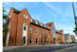
Beaufort House London, UK - 2012 Passive Multiservice
