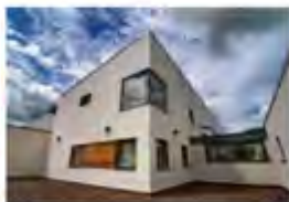
Macmillan Renton Unit Hereford, UK - 2010 Active Chilled Beams
