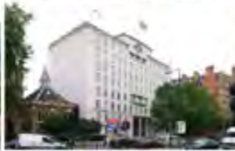
Woolworth House London, UK - 2003 Active Multiservice
