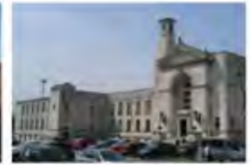
Southampton Civic Centre Southampton UK - 2011 Active Multiservice
