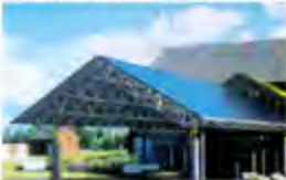
Wrexham A&E Wrexham, UK - 2008 Active Chilled Beams
