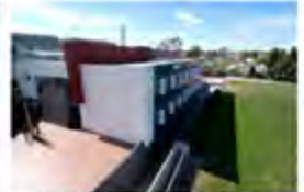
BBC Grafton House Middlesex, UK - 2012 Active Chilled Beams
