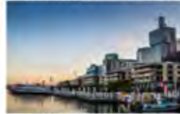
King Street Wharf Australia - 2008 Passive Chilled Beams
