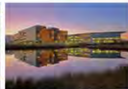
Wollongong University NSW, Australia - 2011 Passive Chilled Beams
