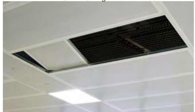
“Hybrid” Radiant / Convective Chilled Beam Ceiling
