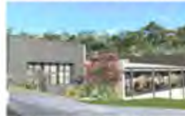
Kingston Aged Care Australia - 2009 Active Chilled Beams
