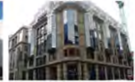
Meridian Court Edinburgh, UK - 2010 Active Chilled Beams
