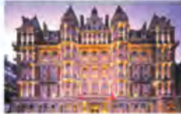
Knightsbridge Hotel London, UK - 2010 Passive Chilled Beams
