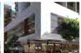
123 Albert Street Brisbane, Australia - 2010 Passive Chilled Beams
