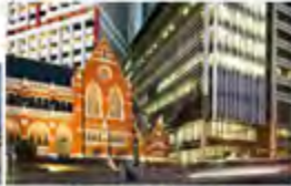
Wesley House Brisbane, Australia - 2008 Passive Chilled Beams
