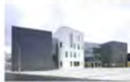
Loxford School London, UK - 2009 Active Chilled Beams
