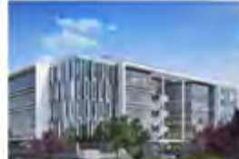
1 Canberra Avenue Australia - 2013 Passive Chilled Beams
