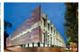
Belconnen Police Australia - 2010 Passive Chilled Beams
