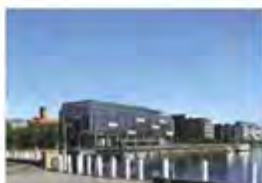
Google Headoffice Sydney, Australia - 2010 Passive Chilled Beams
