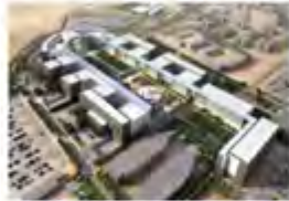
King Saud Bin Abdul Saudi Arabia - 2011 Active Chilled Beams
