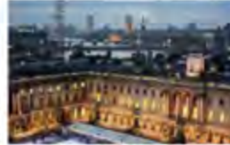
Kings College London, UK - 2009 Passive Chilled Beams
