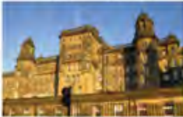
GRI Gynaecology Glasgow, UK - 2008 Active Chilled Beams
