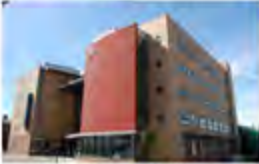
Liverpool College Liverpool, UK - 2010 Active Chilled Beams
