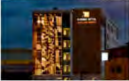
Sudima Hotel New Zealand - 2010 Active Chilled Beams
