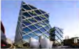
1 Shelly Street Sydney, Australia - 2009 Passive Chilled Beams
