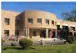
University of Botswana Botswana - 2011 Active Chilled Beams
