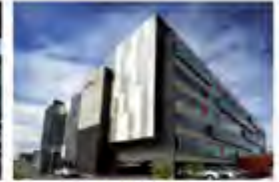
World Park Adelaide, Australia - 2011 Passive Chilled Beams
