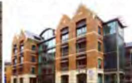
BT Nottingham Nottingham - 1998 Passive Chilled Beams
