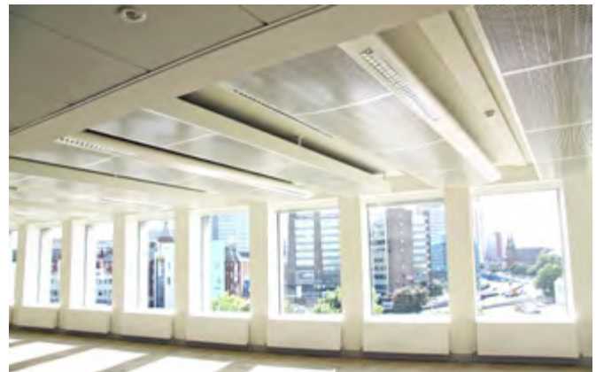
Radiant Passive MSCB
