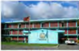
Five Rivers Trinidad - 2010 Passive Chilled Beams
