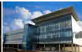
QMC Hospital Nottingham, UK - 2008 Active Chilled Beams
