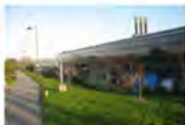
Exeter University Exeter, UK - 2012 Active Chilled Beams
