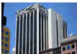
500 Collins Street Australia - 2010 Active Multiservice
