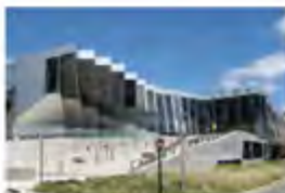
ANU Australia - 2013 Active Chilled Beams
