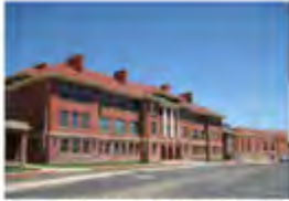
Trinidad School Trinidad & Tobago - 2011 Passive Chilled Beams
