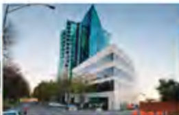
One East Melbourne Victoria, Australia - 2008 Passive Chilled Beams
