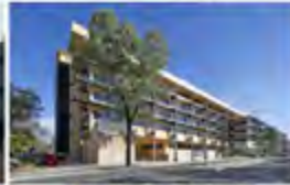
64 Allara Street Australia - 2007 Passive Chilled Beams
