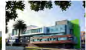
Warnambool Hospital Australia - 2009 Active Chilled Beams
