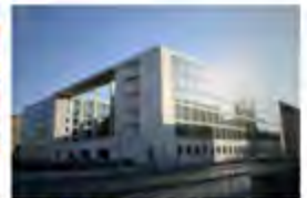
SIEC Tonsley House Australia - 2013 Active & Passive Chilled Beams
