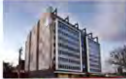
South Australia Police Adelaide, Australia - 2009 Passive Chilled Beams
