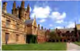
University of Sydney Sydney, Australia - 2007 Passive Chilled Beams
