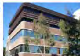
RMIT 9 Australia - 2010 Active Chilled Beams
