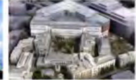
St Barts Hospital London, UK - 2009 Active Chilled Beams
