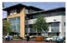
Veolia Environmental Cannock, UK - 2012 Passive Chilled Beams
