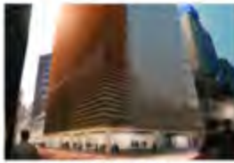
50 Flinders Street Adelaide, Australia - 2014 Passive Chilled Beams
