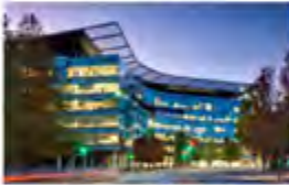
London Circuit Canberra, Australia - 2006 Passive Chilled Beams
