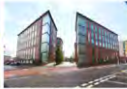
Langley Point Birmingham, UK - 2012 Passive Chilled Beams
